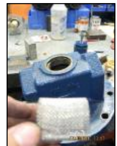
Remove, inspect and clean strainer.
